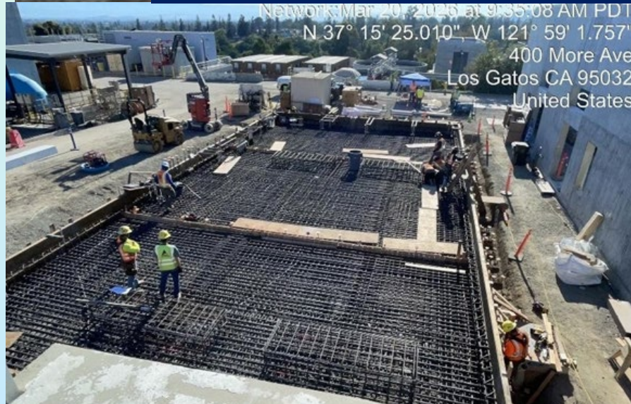
Foundation Slab Rebar
