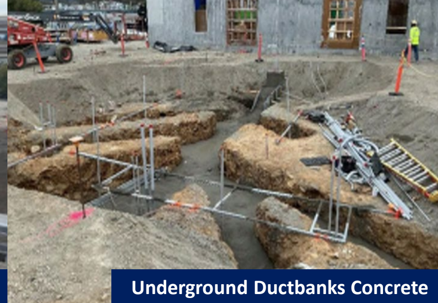
Underground Ductbanks Excavation
