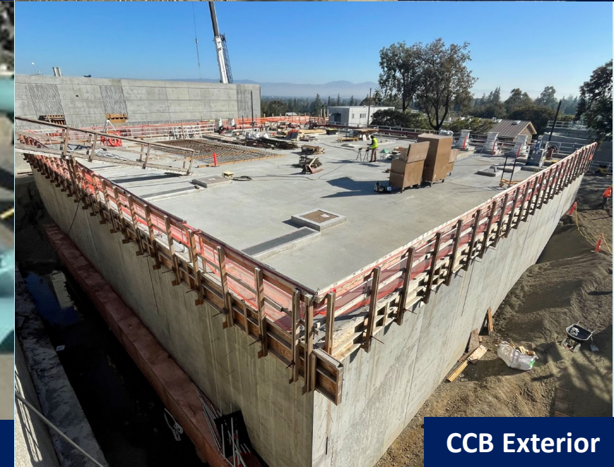
Deck Handrails
